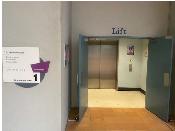
Level 1 - Lift #11 (Access point for access to go to level 3)
